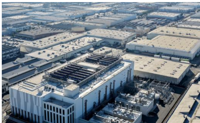
An aerial view of a 33 megawatt data center (LOWER L) with closed-loop cooling system, amid warehouses on October 20, 2025 in Vernon, California. A surge in demand for AI infrastructure is fueling a boom in data centers across the country and around the globe. Source: Salon
