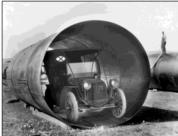
Image 1 Automobile inside steel siphon pipe
